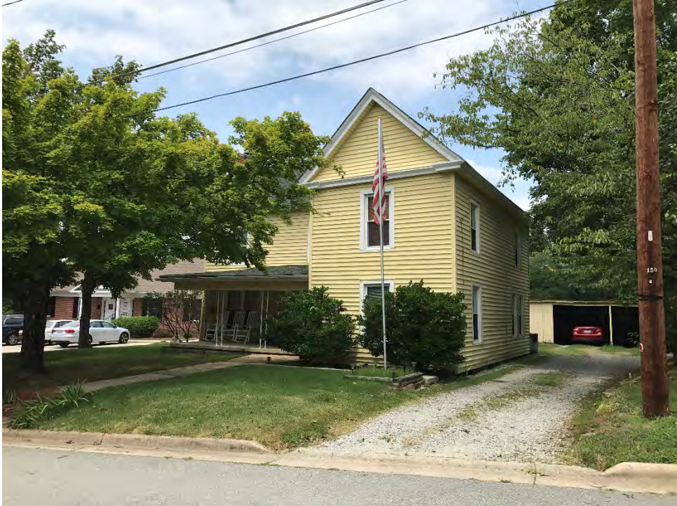
211 OAKDALE RD – Built 1887
