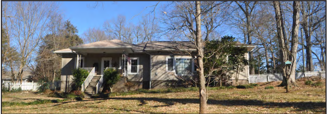
A. Southwest Side
