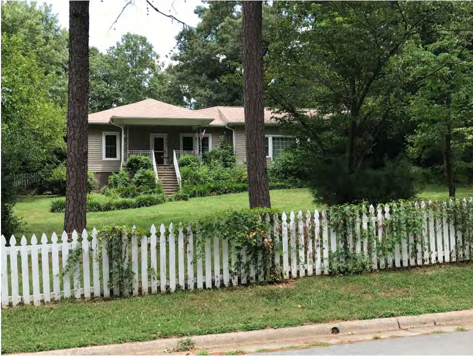
301 OAKDALE RD – Built 1929
