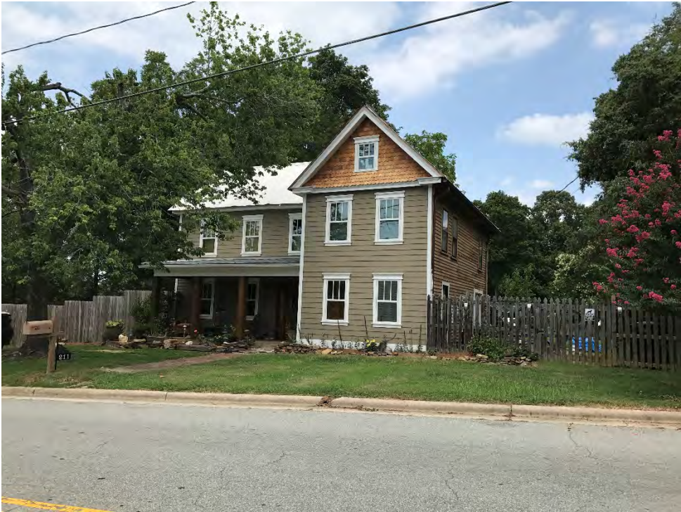
303 OAKDALE RD – Built 1918
