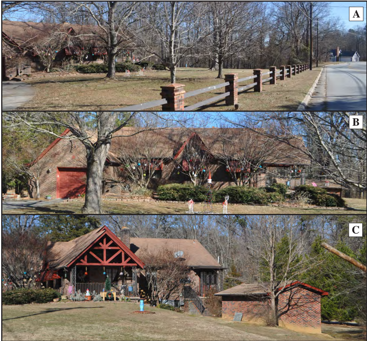
A. Perimeter Fence on Oakdale Road; B. West Side; C. South Side with Outbuilding and Abandoned Driveway
