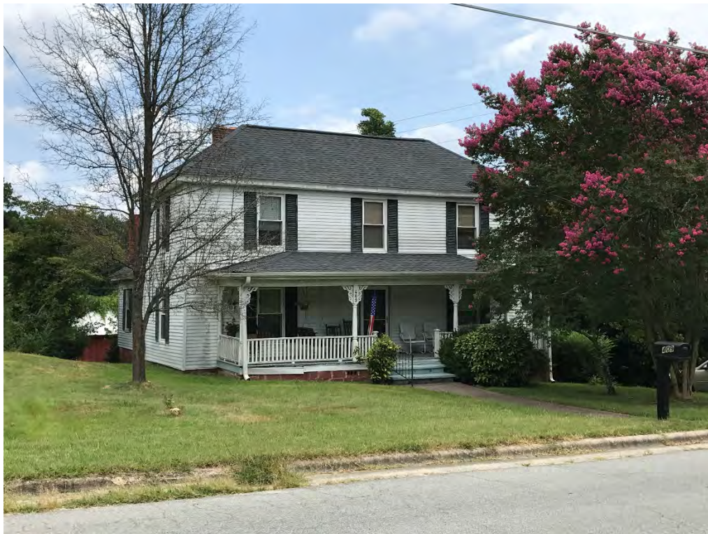
505 OAKDALE RD – Built 1948
