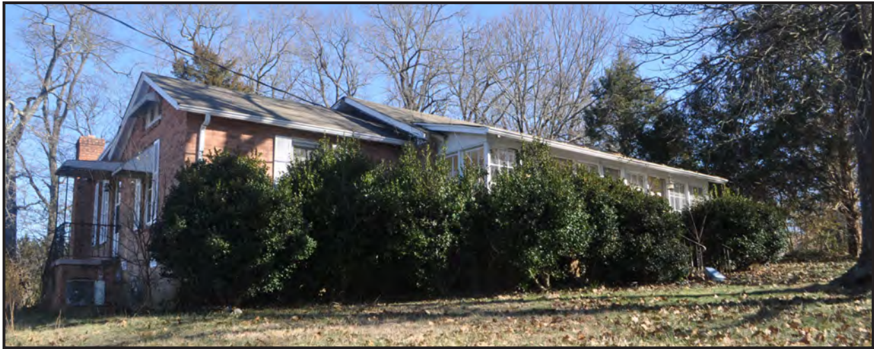
A. Southwest Side And Section Of Stone Wall
